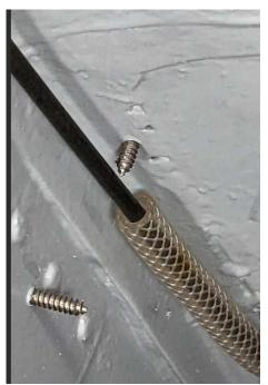
For instance, this first test hole was offset but a check showed that a vibrating line near sharp screws is asking for trouble.
