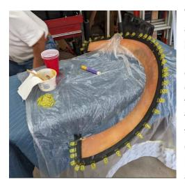
While all the above is taking place, the flare has been getting a custom rubber flange carefully fitted and glued to the edge, clamped tightly in place all along the edge
