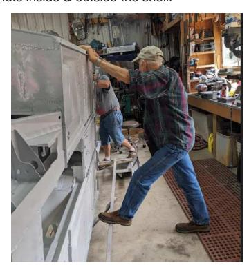
Use heavy-duty sawhorses covered with cloth to hold the shell for mounting parts.
