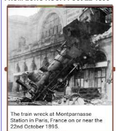
No. 56, arriving from Grandville, at 40-60 KM, was unable to stop, ploughed through the station buffers, across 30 metres (98 ft) of the concourse to the end of the platform, crashed through the 24 " thick station building façade wall, and fell nose down onto Place de Rennes, killing a newspaper seller Marie-Augustine Aguillard.
